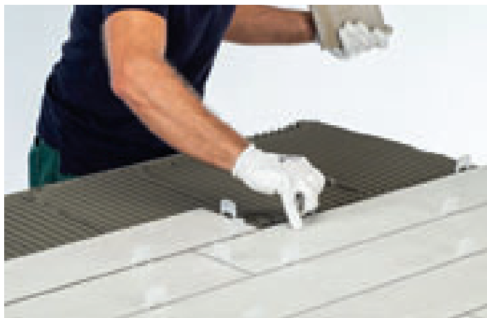
disposable clips installation
